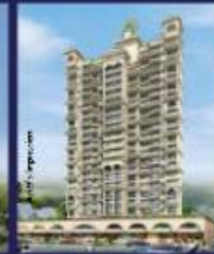
SAI MOKSH KHARGHAR G+22 Storeyed Tower
