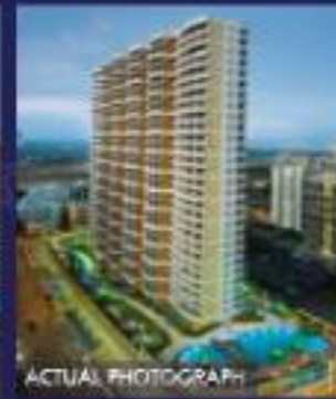
SAI CRYSTALS KHARGHAR G+30 Storeyed Tower with 2 Wings
