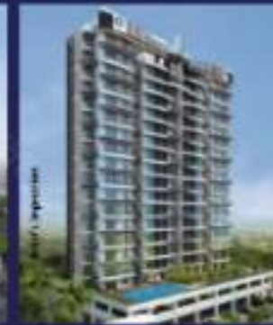
SAI WONDER KHARGHAR G+18 Storeyed Tower
