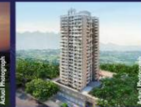
SAI AARADHYA KHARGHAR G+22 Storeyed Tower
