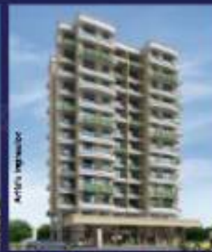
SAI SAHIL ULWE G+12 Storeyed Tower
