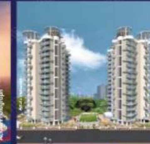
SAI PEARLS KHARGHAR G+15 Storeyed 2 Towers
