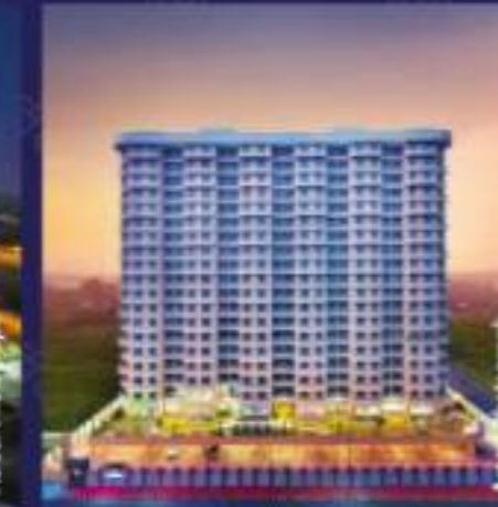
SAI RIVERDALE TALAJA G+19 Storeyed Tower with 2 Wings
